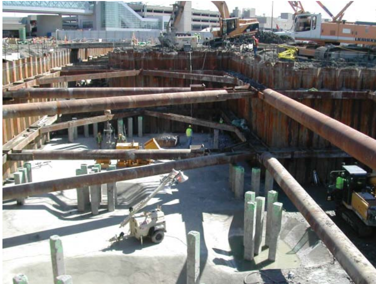
Fig. 7.3 Braced sheet pile wall. (Photo courtesy of Earthwork Engineering, Inc. Hollis, New Hampshire.)
