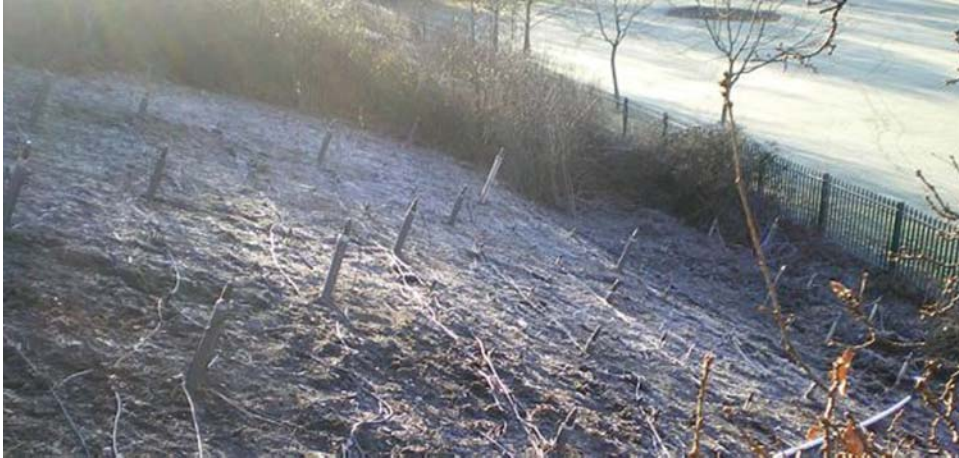
Fig. 6.10 A field project using electroosmosis. (Photo courtesy of Electrokinetic Limited, UK.)
