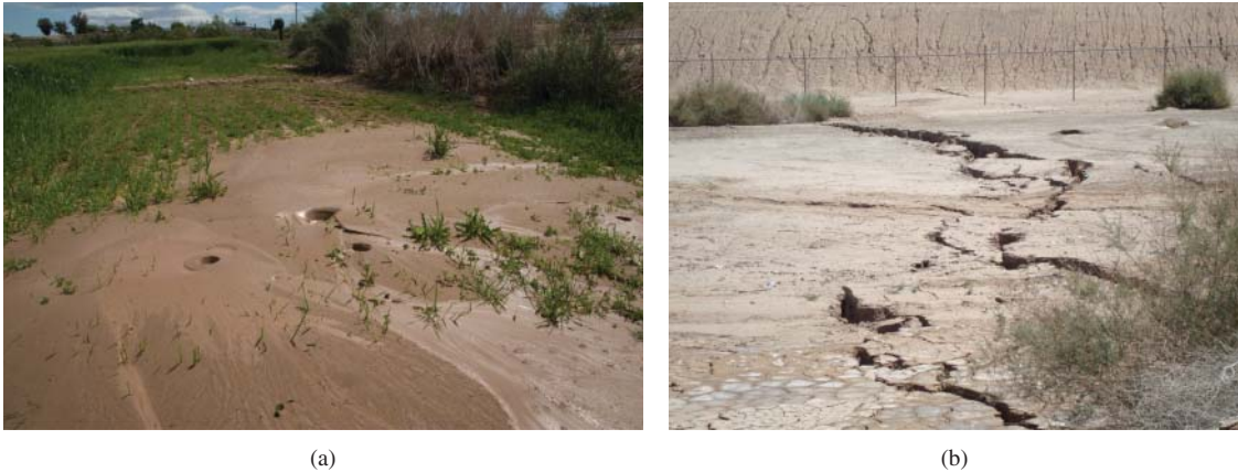
Fig. 9.21 Liquefaction in the 2010 Baja California earthquake ( M_w = 7.2 ). (a) Sand boil (Photo courtesy of Prof. Scott J. Brandenburg, University of California, Los Angeles.), (b) Land lateral spread because of liquefaction. (Photo courtesy of Timothy P. McCrink, California Geological Survey.)
