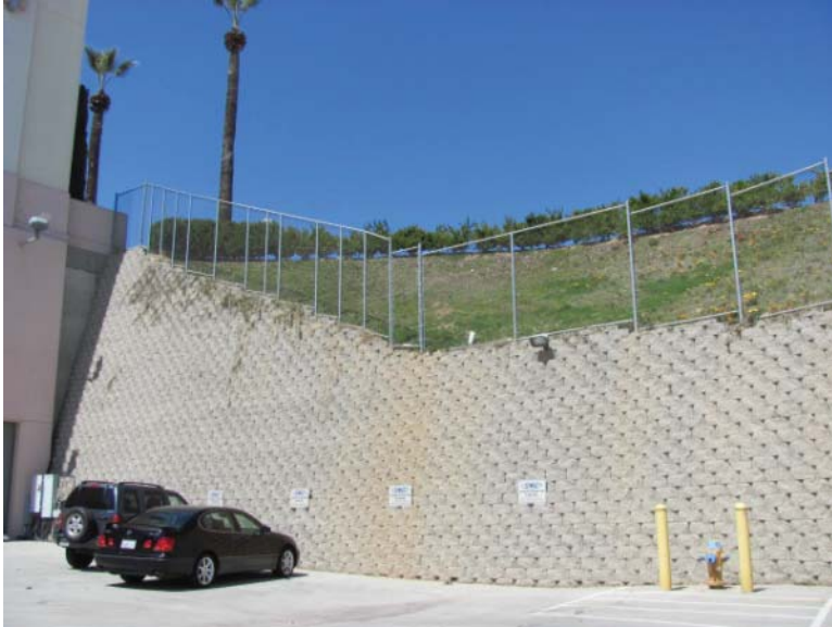
Fig. 7.1 Retaining wall on the campus of California State University, Fresno, USA.
