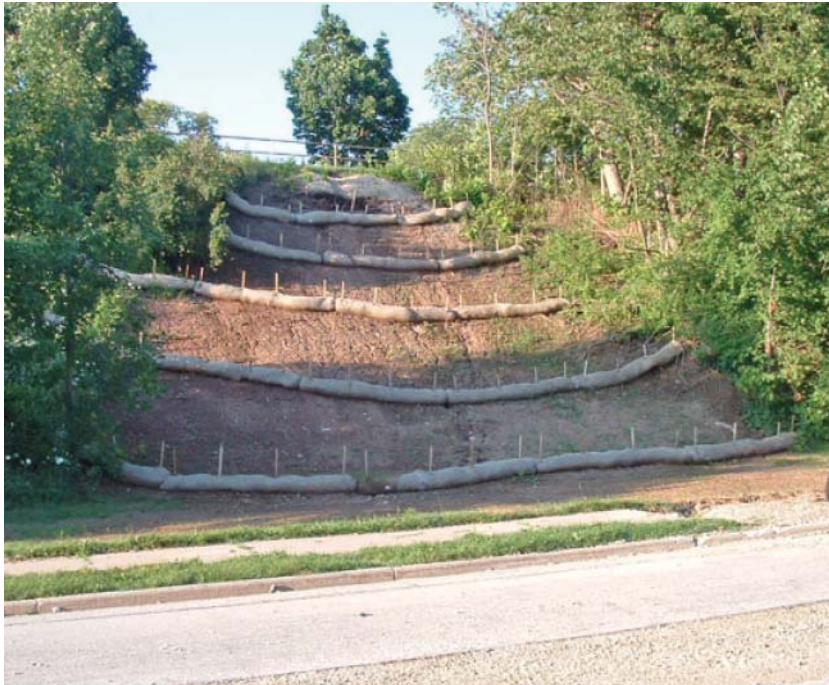
Fig. 5.28 Surface erosion control using straw tubes.
